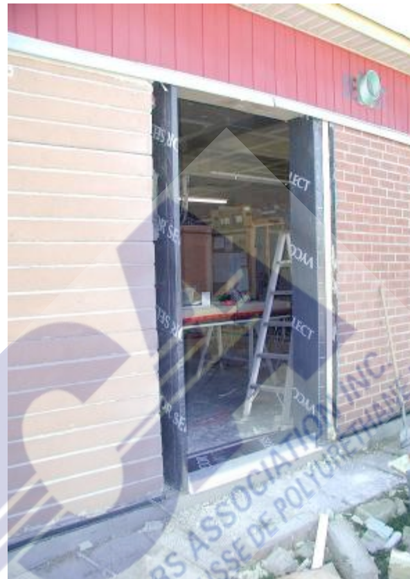
Figure 2.2: Opening perimeter details for removable test walls
